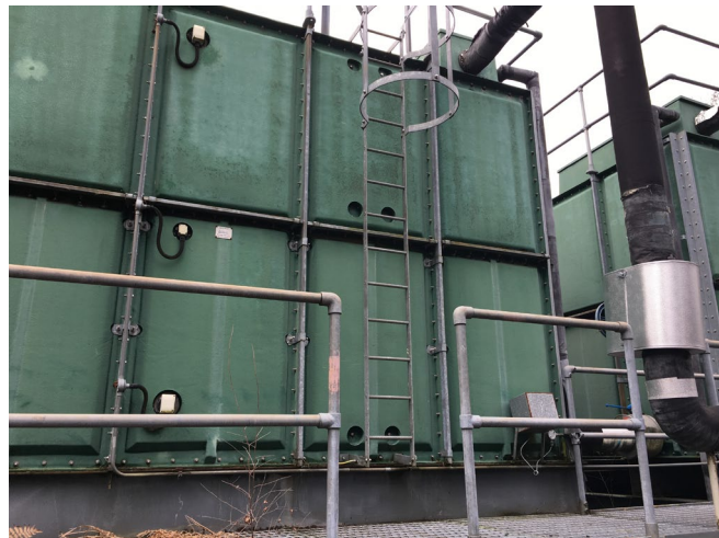
External view of Tank 1
