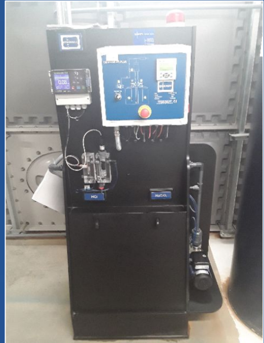
One of the Chlorine Dioxide systems treating one of the massive 136,000 lts CWS tank
