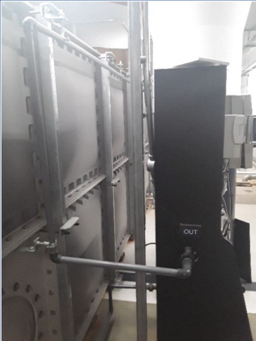
One of the Chlorine Dioxide systems treating one of the massive 136,000 lts CWS tank
