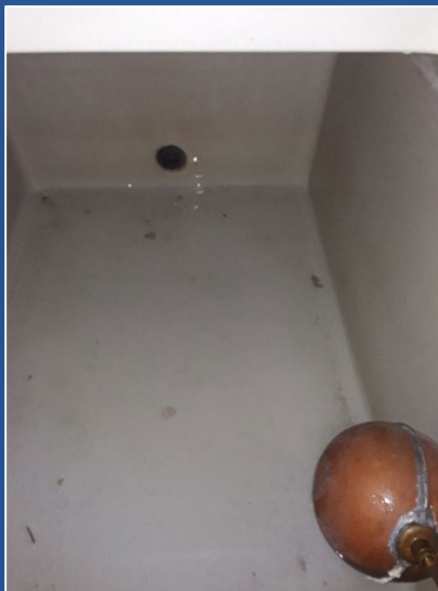
Tank internal – After cleaning
