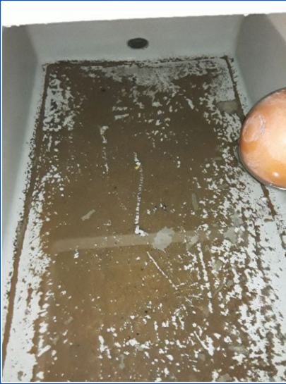
Tank internal – Before cleaning
